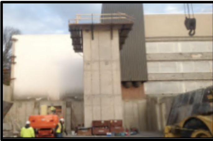
Figure 1 Installation of Stair Tower A
